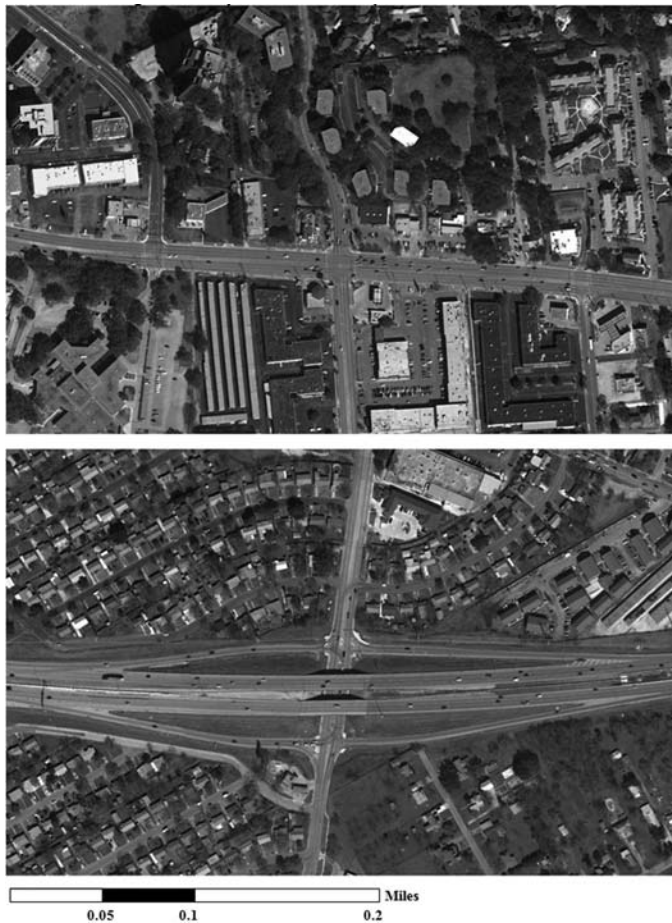
Figure 7. Unlike arterials (top), freeways (bottom) are designed to eliminate the traffic conflicts occurring at driveways and intersections.
